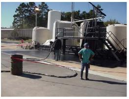
The project specification called for blast cleaning of the concrete pit area and steel walkway structure. The pit area had a small berm wall surrounding the pit to trap any spills or leakage. A 1/4" key way was cut around the berm perimeter to allow for lock-in of the PCS-325 system. After preparation, the area was primed using the DURA-PLATE 235 epoxy processed through airless spray equipment at a thickness of 8—10 mils. Some back-rolling was also required.
