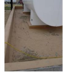
After over 1 year of service, the applied FSS 45DC SS aromatic polyurea elastomer system (beige) is performing well. While there have
