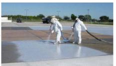
was experiencing severe cracking and concerns were had over potential spills of fuel seeping into the ground water. The PV 350 polyurea system was chosen due to excellent performance history in similar application areas, flexibility, toughness for heavy traffic and speed of installation.
