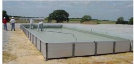
BBL Falcon Industries has a patent pending procedure for rehabilitating existing tank drilling sites, as well as new installation areas. Designed areas are cleaned and leveled, the metal perimeter installed and the geo-textile fabric laid. The FSS-45DC applied up and onto the geotextile and perimeter wall area. Once laid in place and sprayed with the FSS-45DC up and onto the perimeter wall, the tanks and piping are set in place.
